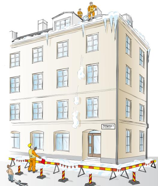
**"The man in the street"** is to be equipped with protective helmet, high-vis jacket and signalling device as well as communication equipment to the workers on the roof, a whistle, siren or telephone.
