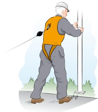
There may be risk of stepping through surfaces whose load-bearing capacity is inadequate and such areas should be cordoned off. Use special safety equipment if work shall nevertheless be performed on such a surface.
